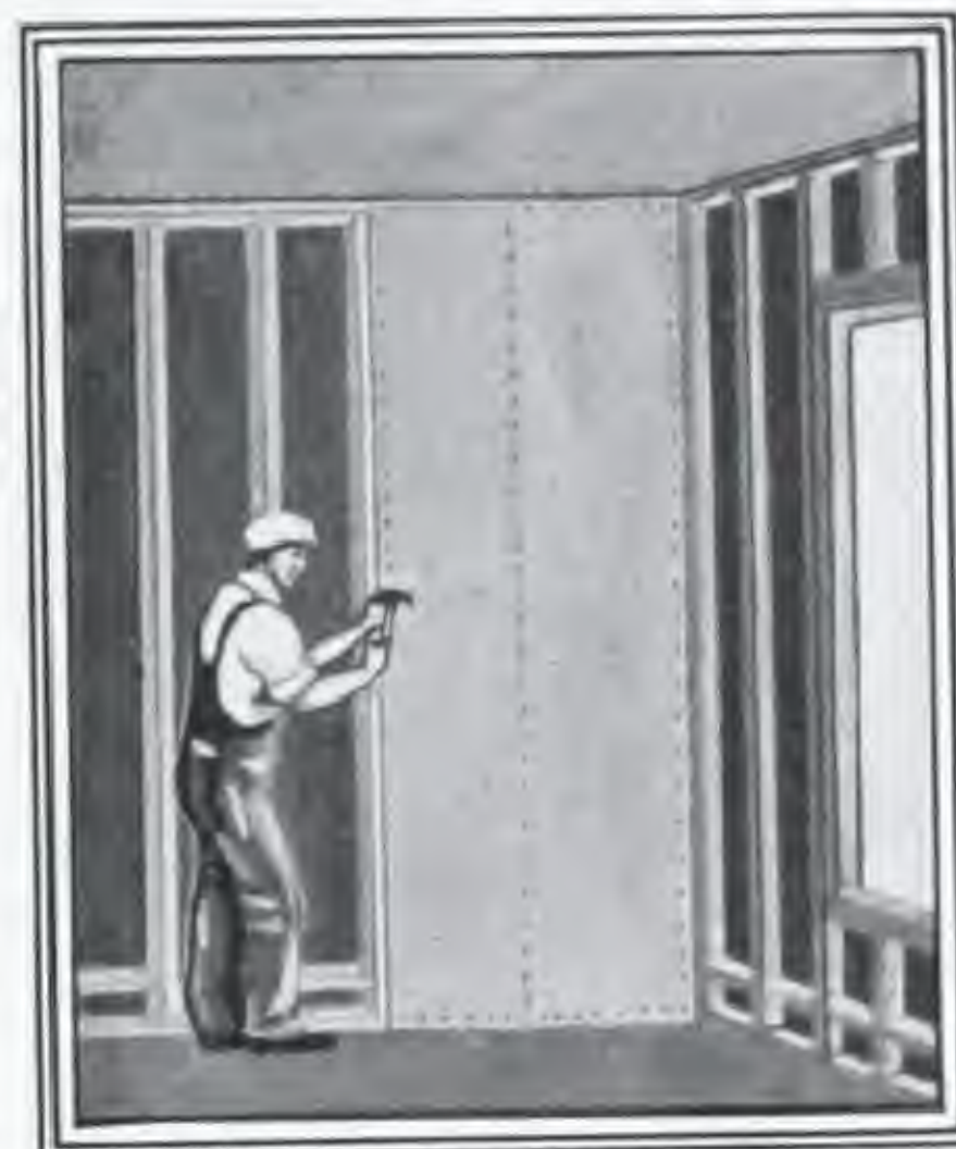
APPLYING GYPROC WALL BOARD
