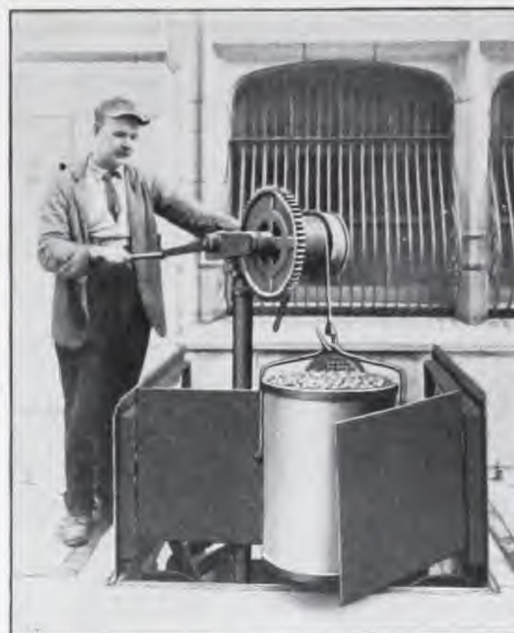
FIG. 6. MODEL A. REVOLVING HOISTING HEAD WITH CAN.
