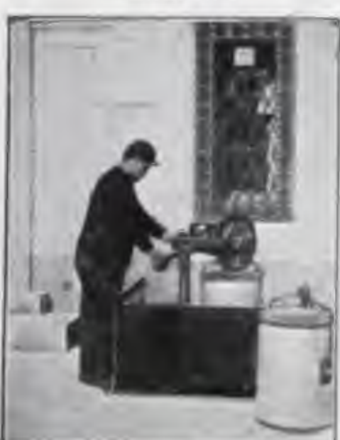
Lowering empty cans. Hoisting handle does not revolve.
