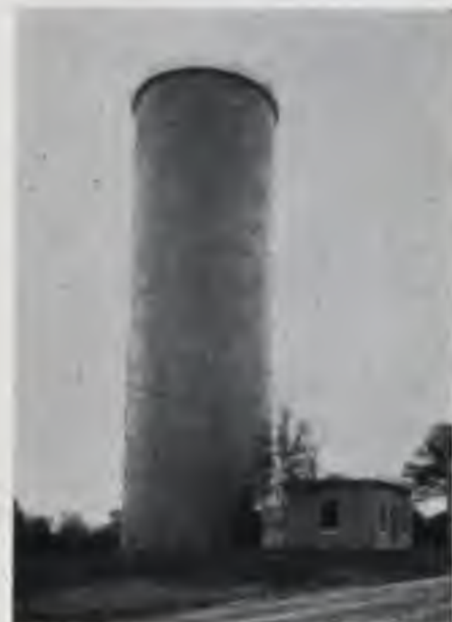
STEEL STANDPIPE, MUNICIPAL WATERWORKS.
