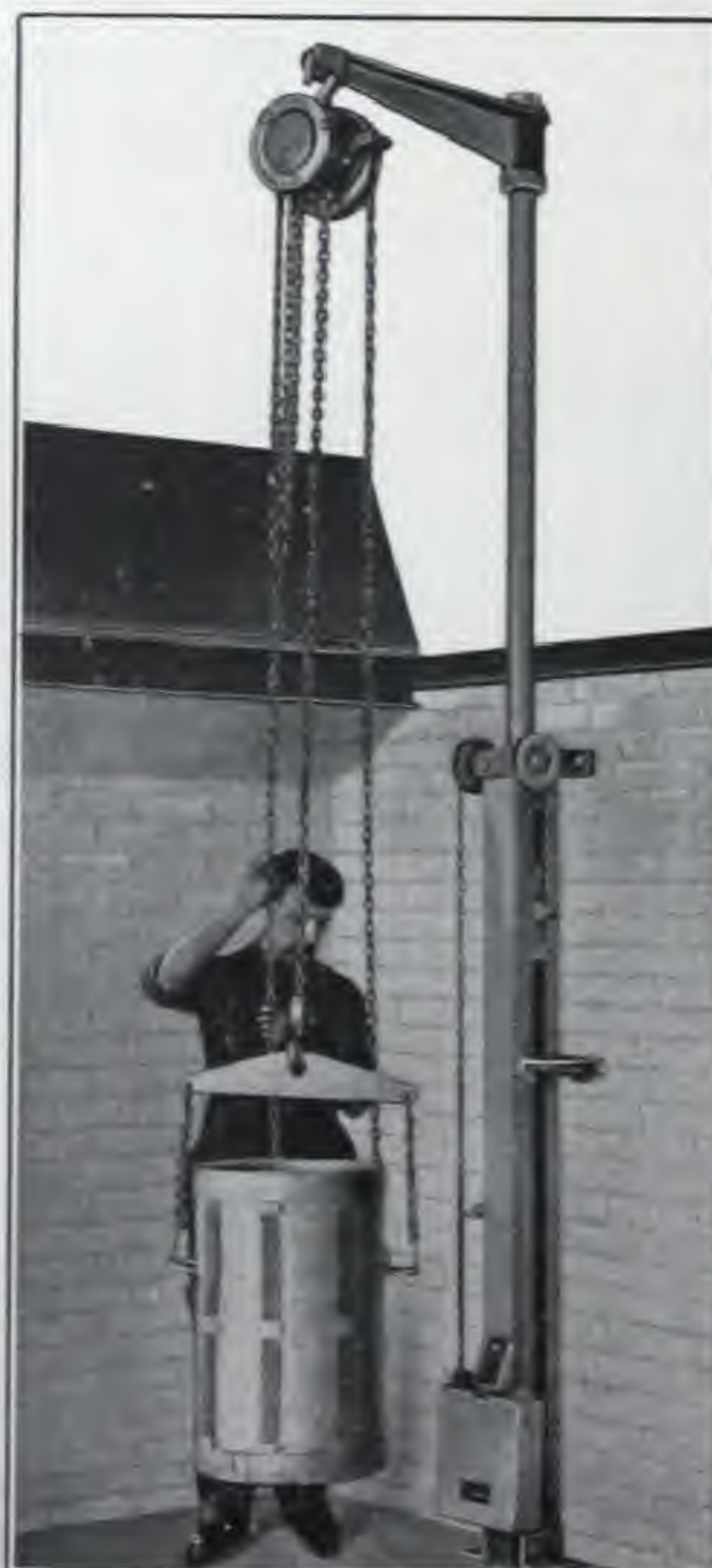
B. 404. TELESCOPIC ASH-HOIST.
