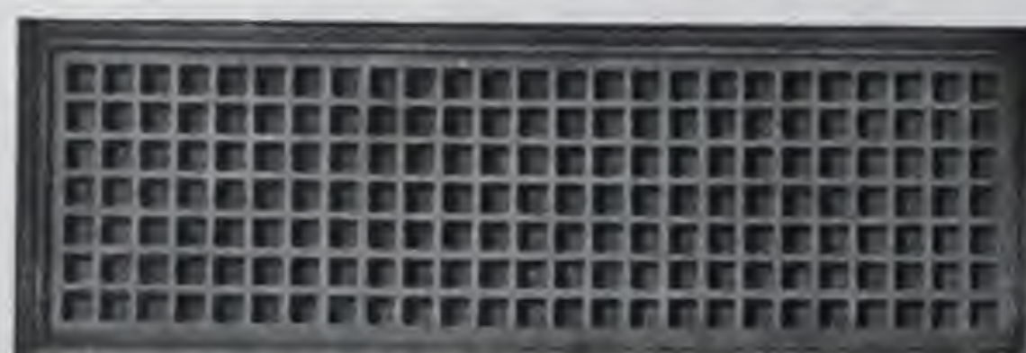
GRILLE HELD IN PLACE BY WOOD MOULDING.
