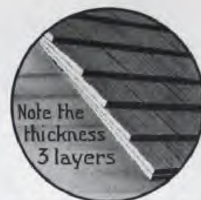
THE PROPERLY LAID SHINGLE ROOF —GOOD FOR A GENERATION OF SATISFACTORY SERVICE.
