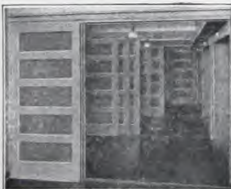
PARALLEL PARTITIONS. Hung on trolley track for combining several small rooms into one large room in schools, churches and auditoriums.
