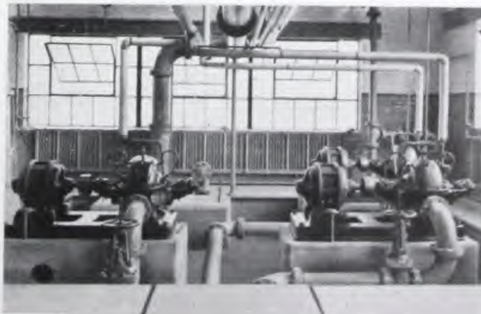
3 REES-RO-TURBO CIRCULATING PUMPS RECENTLY INSTALLED AT THE PLANT OF THE LOG SUPPLY CO., BERTHOE, QUE.
