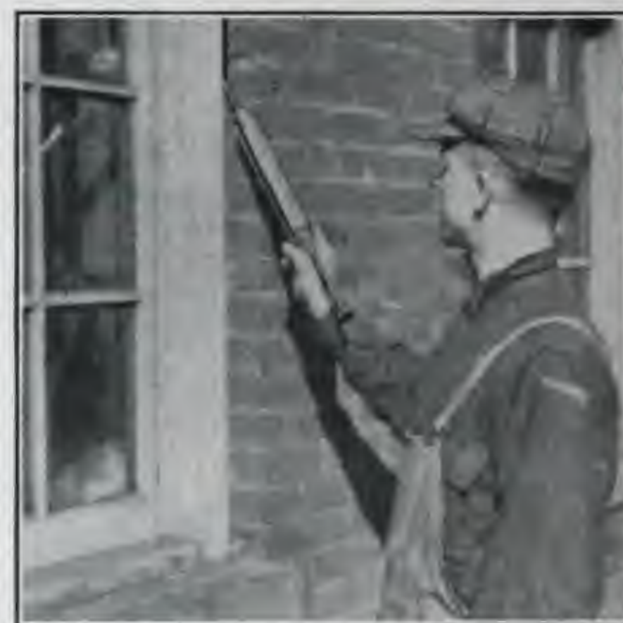
CAULKING AROUND WINDOW FRAMES.
