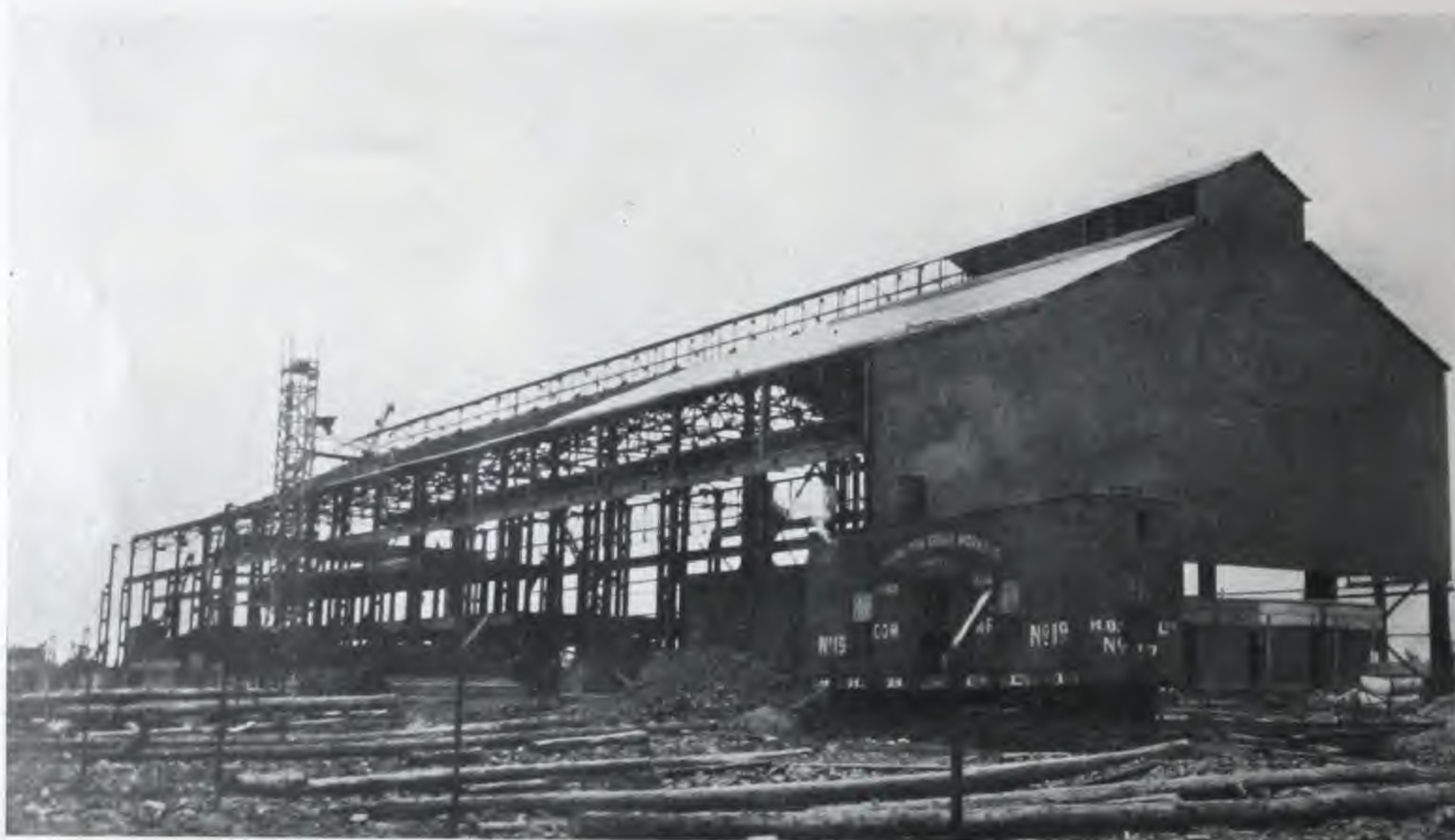
STRUCTURAL STEEL MILL BUILDING, RECENTLY FABRICATED AND ERECTED BY HAMILTON BRIDGE WORKS CO., LIMITED.
