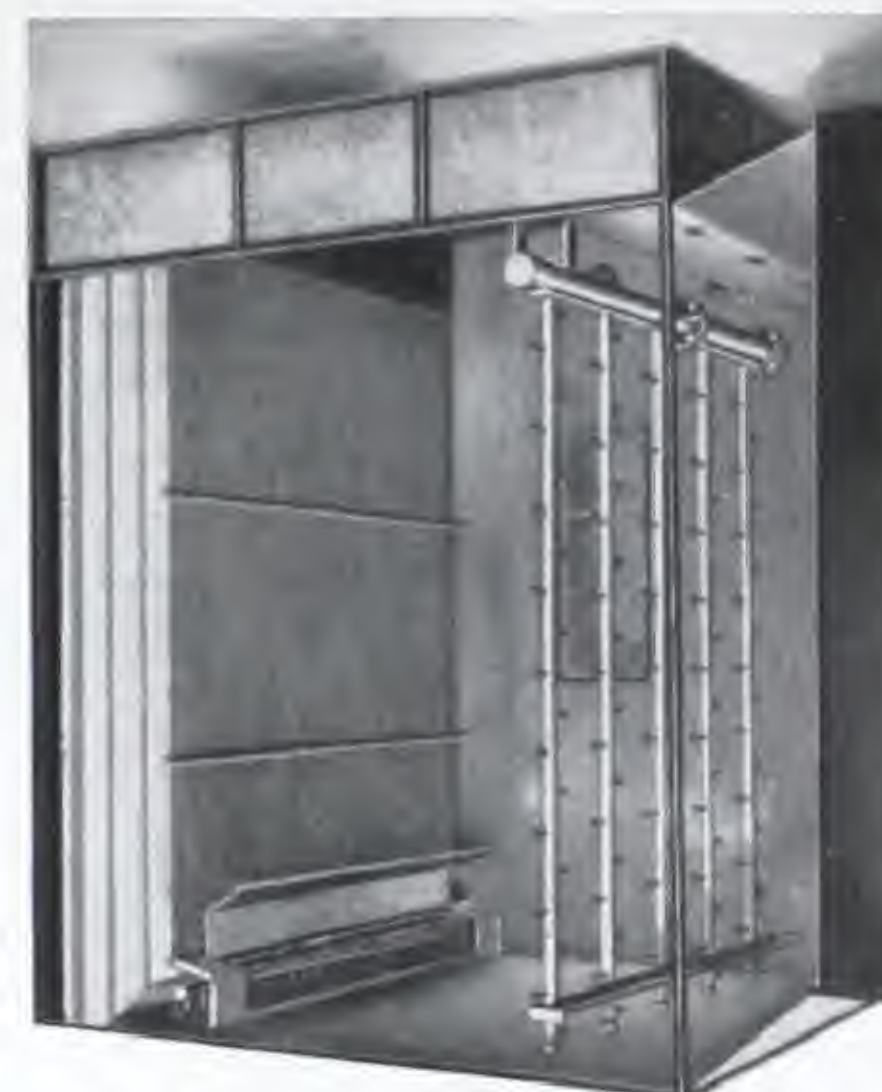
INTERIOR CARRIER AIR WASHER.
