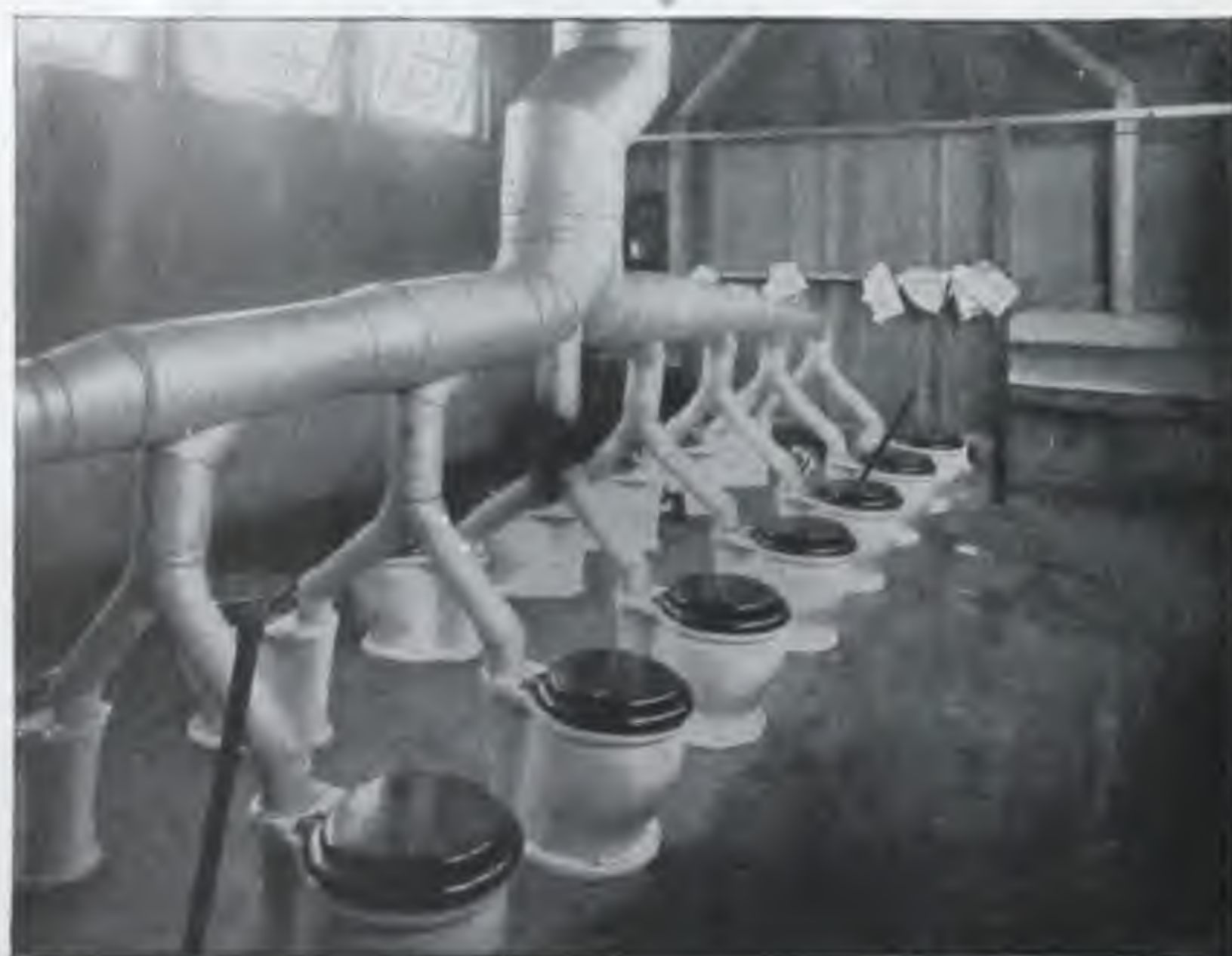
SET UP IN A LARGE TORONTO INDUSTRIAL PLANT, SHOWING VENT PIPE BEFORE BEING COVERED IN.
