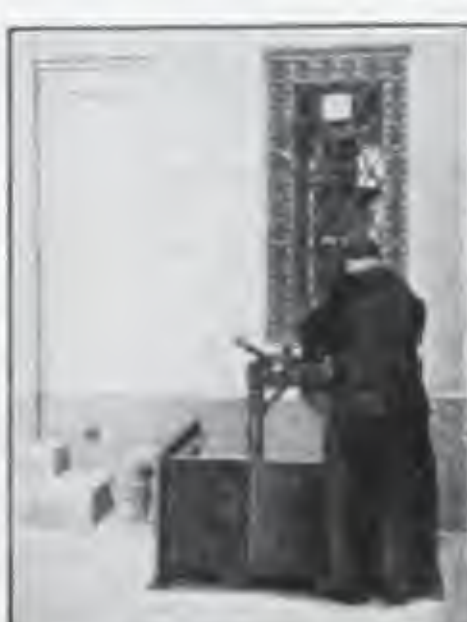
"Hooking" a G & G Standard Hoisting Can with Swing Bail.
