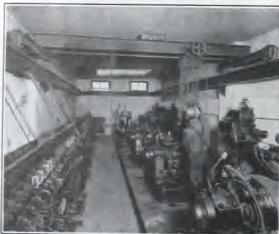
B. 403. SINGLE-BEAM HAND-CRANE
