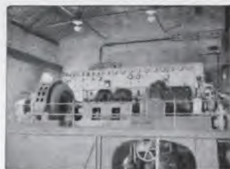
1200 KW. GEARED-TURBINE-DRIVEN ALTERNATOR INSTALLED AT TORONTO.
