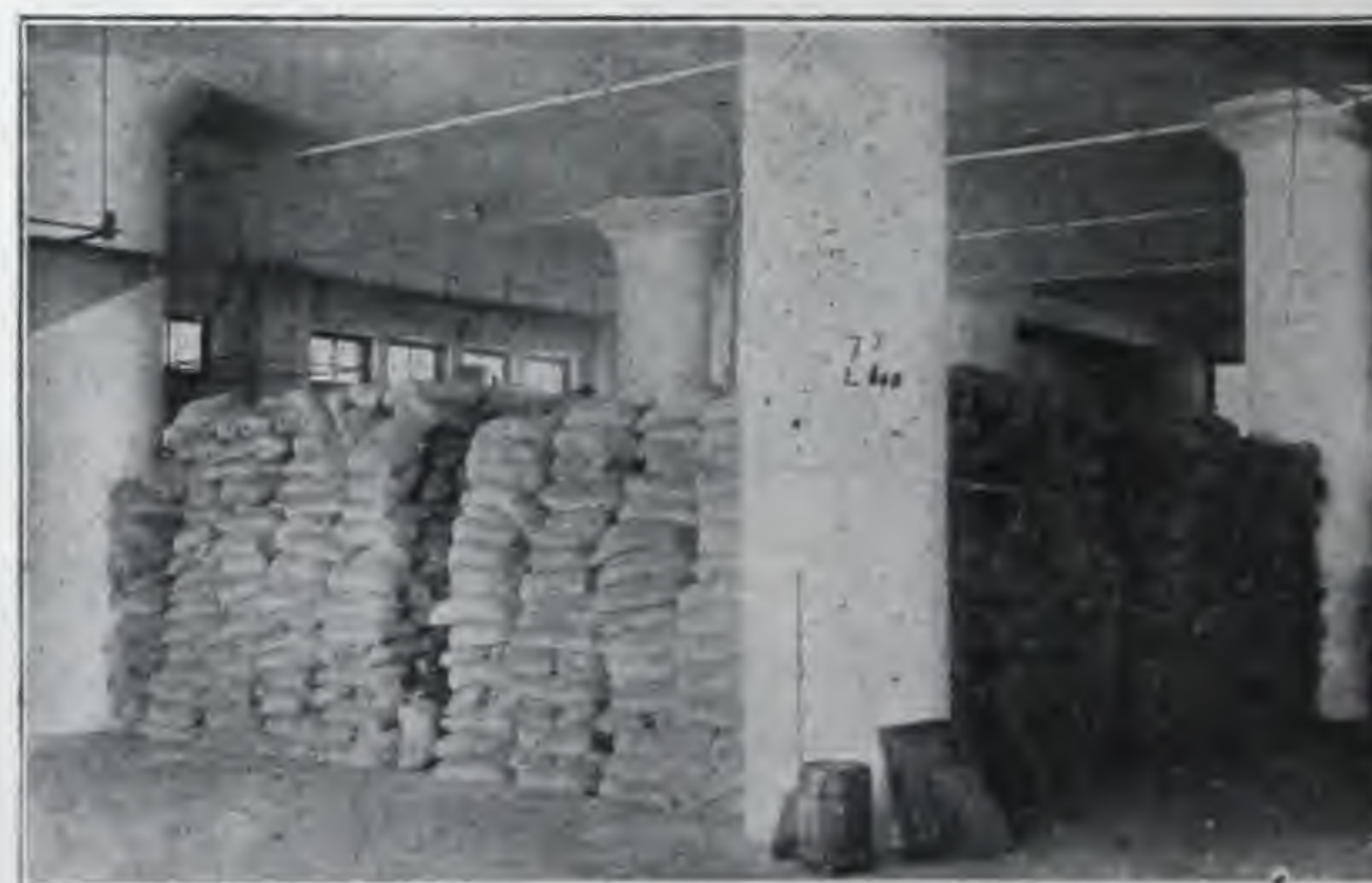
TEST LOAD, 600 LBS. PER SQUARE FOOT. DEFLECTION, \frac{1}{8} INCH
