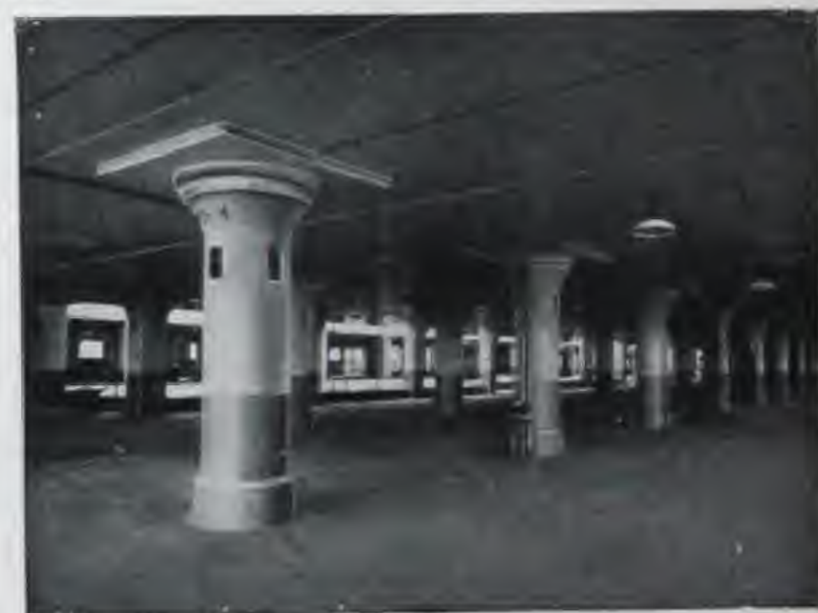
CONCRETE COLUMNS USED AS DISTRIBUTING DUCTS.
