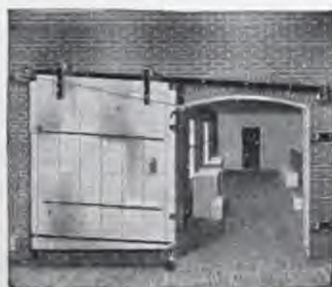
"CROWN" TIN-CLAD FIRE DOORS are made in all styles, and carry the Fire Underwriters' Label.
