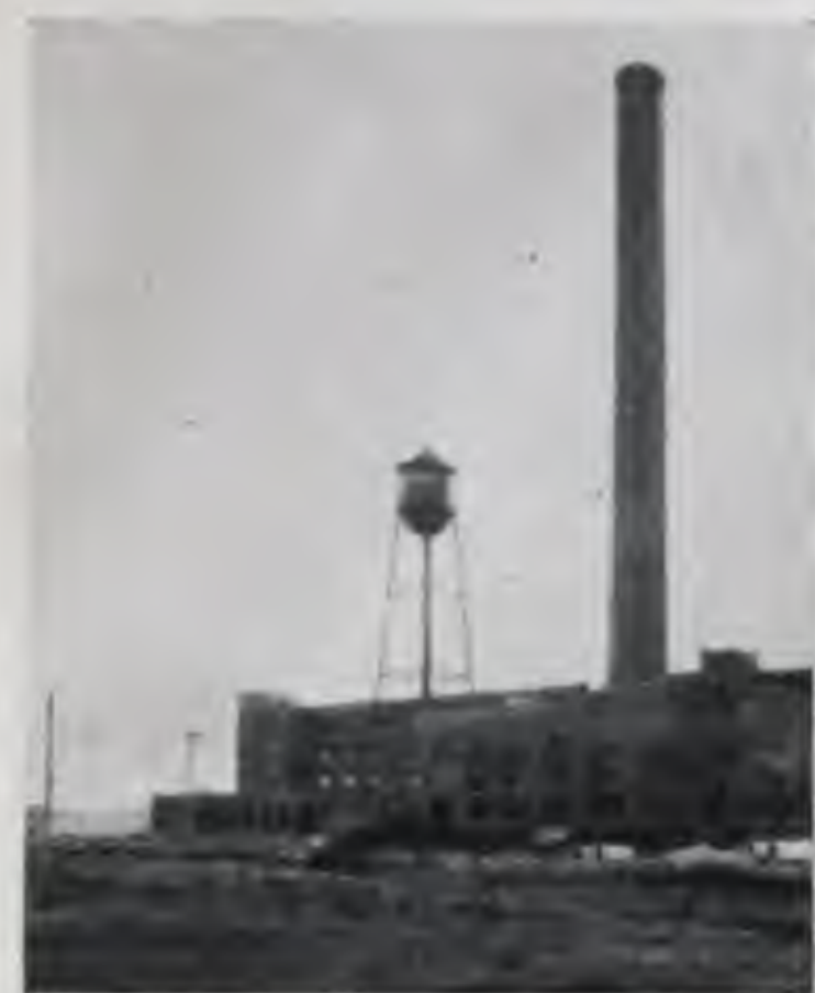
STEEL SPRINKLER TANK FOR INDUSTRIAL PROTECTION.
