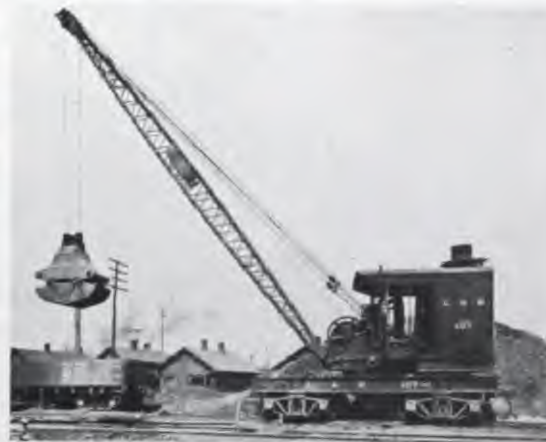
BROWNHOIST No. 4 STEAM LOCOMOTIVE CRANE, EQUIPPED WITH BROWNHOIST 54 CU. FT. COAL GRAB BUCKET.
