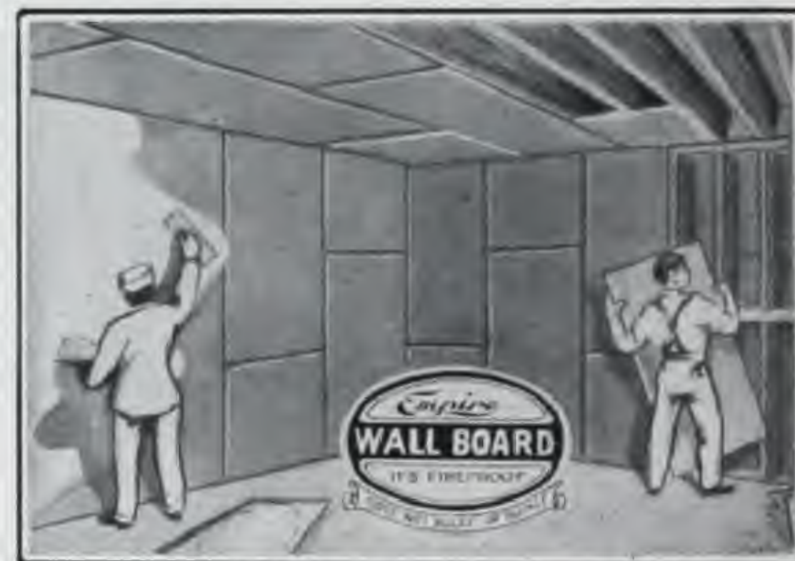
USED AS A BASE FOR HARDWALL OR WOOD FIBRE PLASTER.
