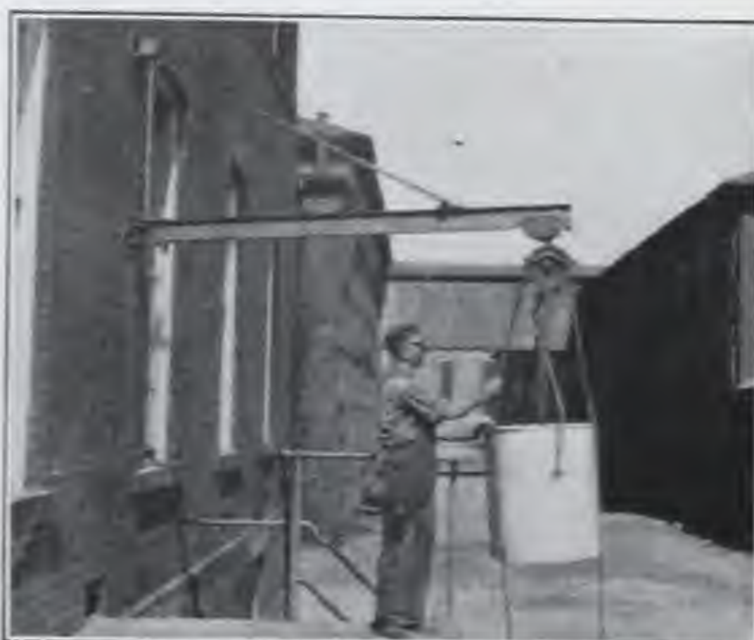
B. 406. WALL-TYPE JIB-CRANE.
