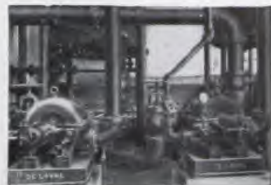
SINGLE-STAGE CIRCULATING PUMPS IN CONNE- CTION WITH HOT-WATER HEATING SYSTEM
