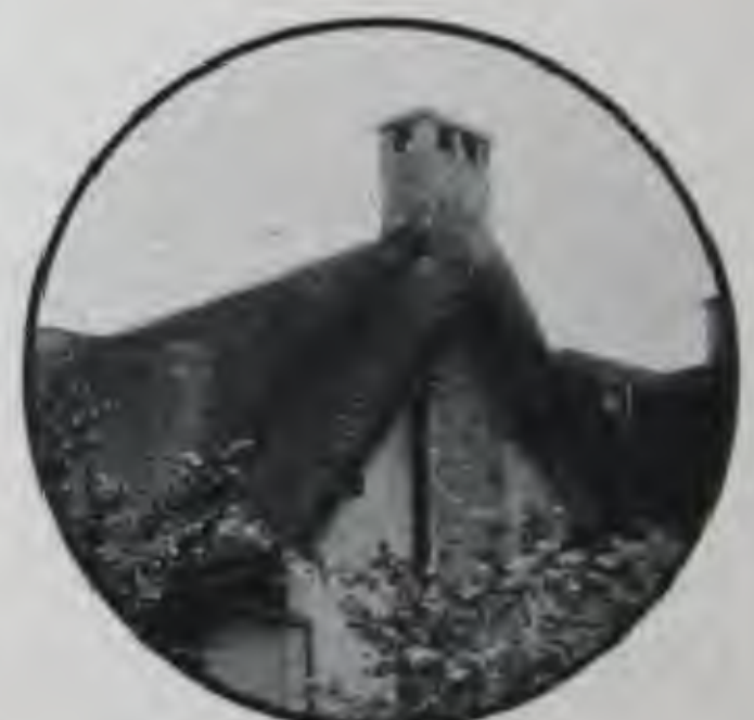
A "THATCHED" SHINGLE ROOF.
