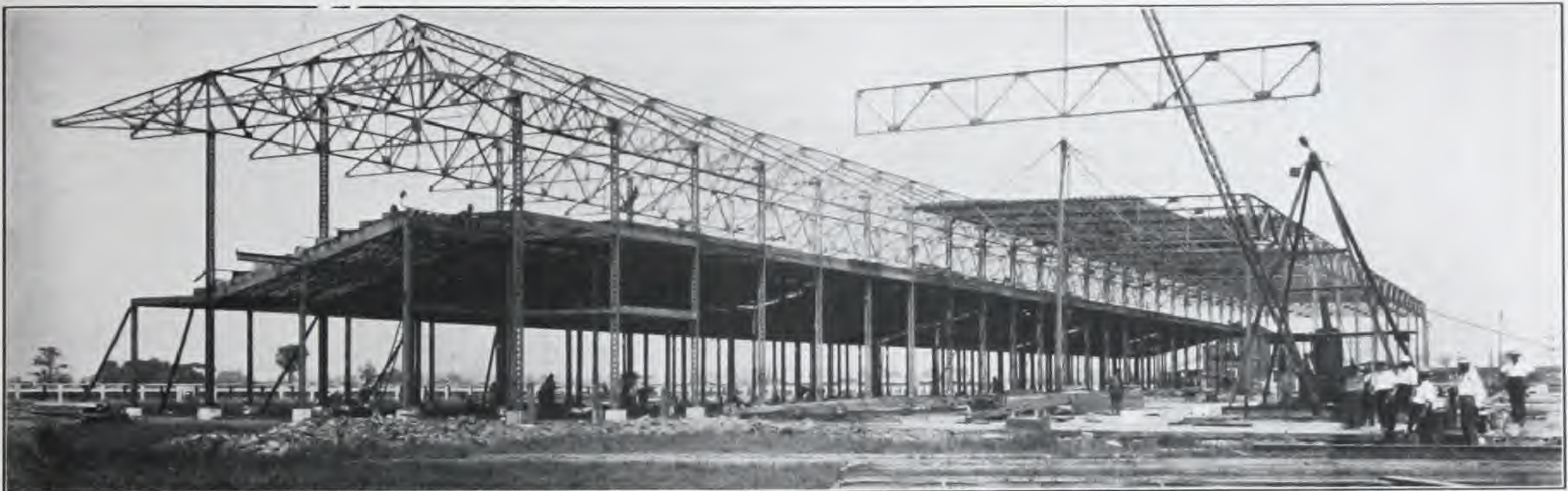
GRAND STAND, 416 ft. Long x 56 ft. Wide. BETTING SHED, 416 ft. Long x 100 ft. Wide x 30 ft. High. Structural Steel Fabricated and Erected by Us in Record Time.
