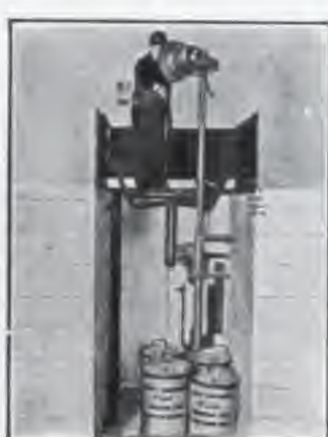
"Hooking" a G & G Standard Hoisting Can with Swing Bail.
