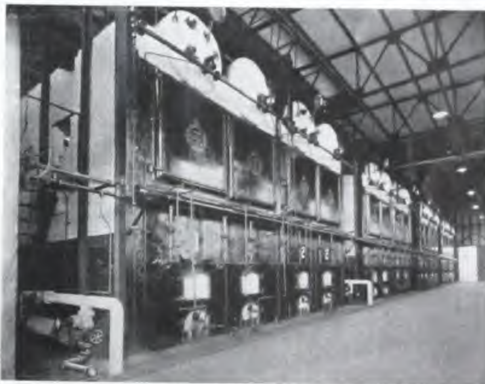
A RECENT INSTALLATION OF 8 DOUBLE DRUM G. & McC. SECTIONAL WATER TUBE BOILERS AT THE DARTMOUTH, N.S., PLANT OF THE IMPERIAL OIL CO.
