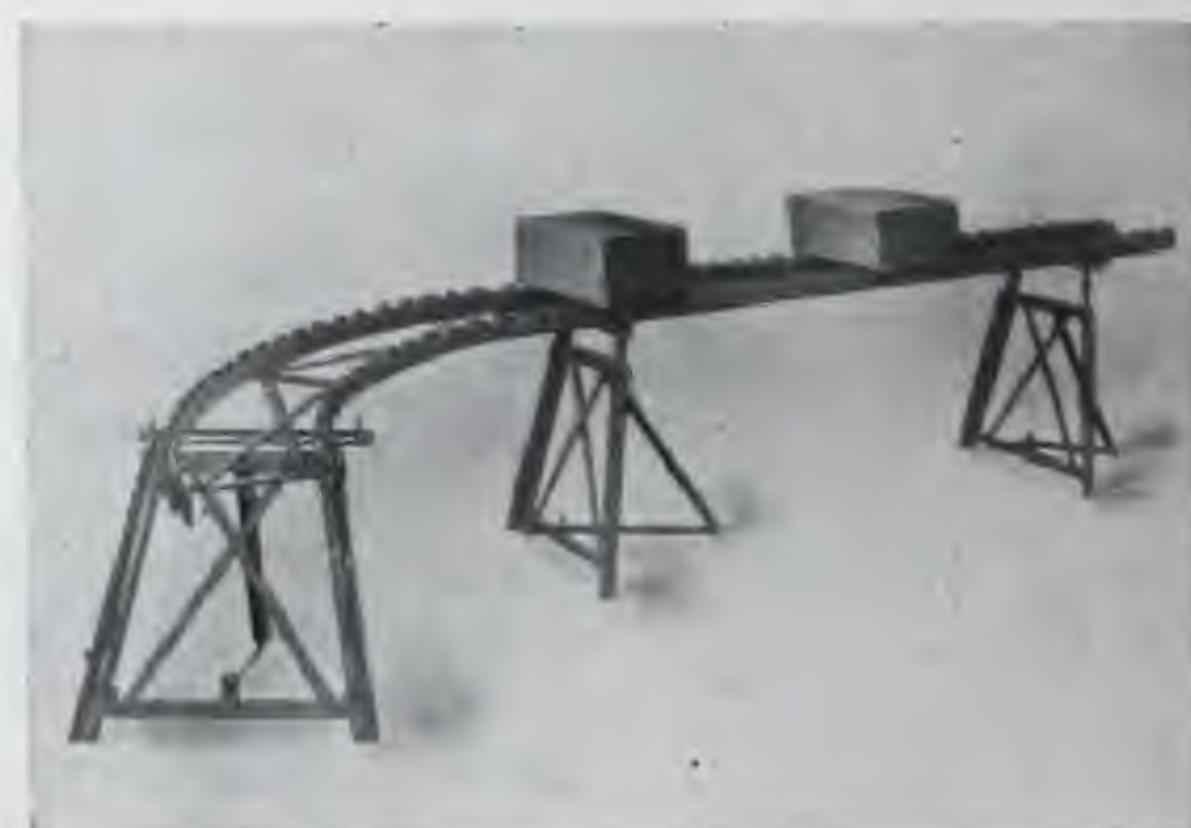
GRAVITY WHEEL CONVEYOR.
