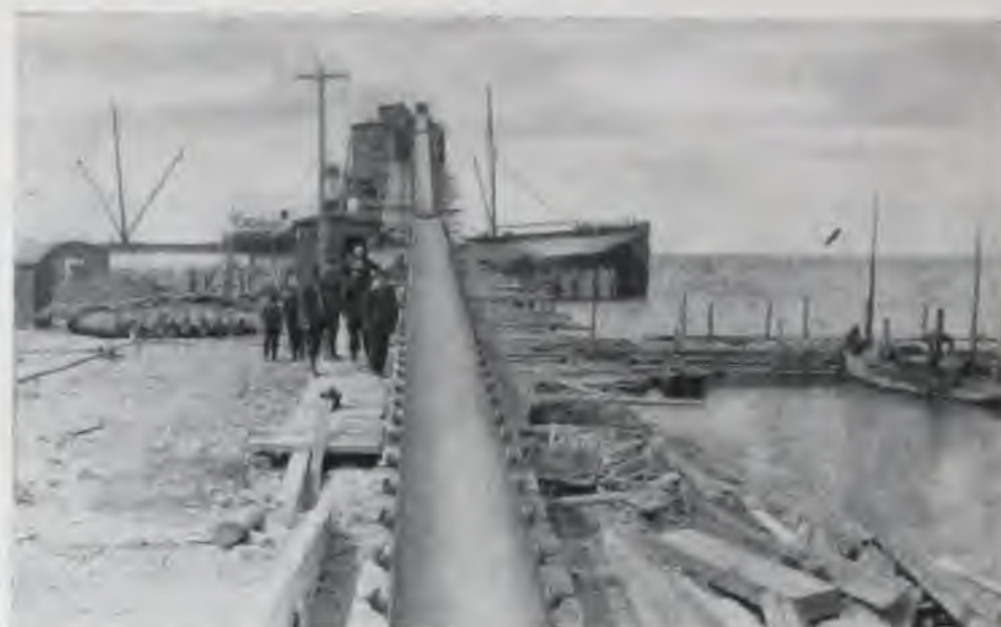
Loading dock at the limestone quarry of the Dominion Iron & Steel Company, Port au Port, Newfoundland, where Robins Conveying Machinery is used to put limestone into and carry it away from storage, and finally load it into ships.
