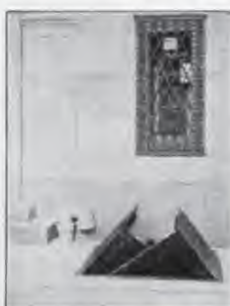
As hoisting head is lowered, doors automatically close.
