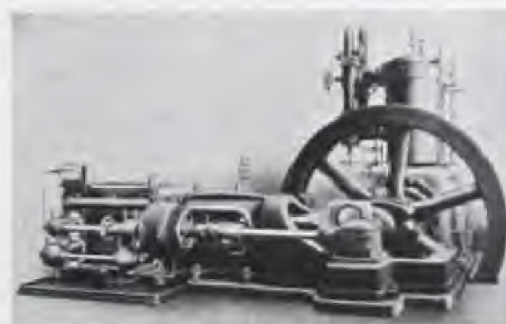
VERTICAL HIGH SPEED COMPRESSOR WITH UNIFLOW ENGINE.
