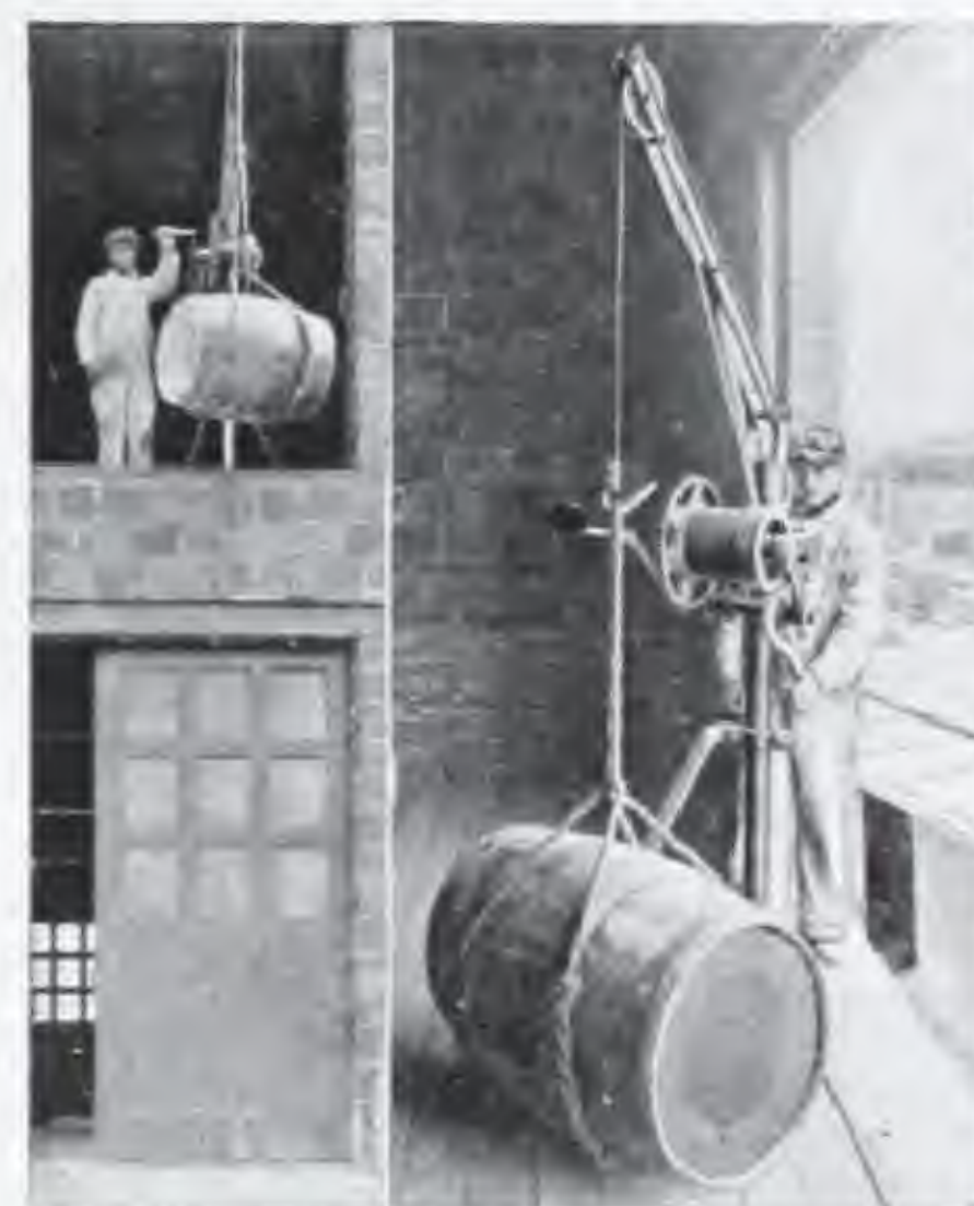
FIG. 8. MODEL B. NON-TELESCOPIC HOIST AS USED IN A CHEMICAL PLANT.
