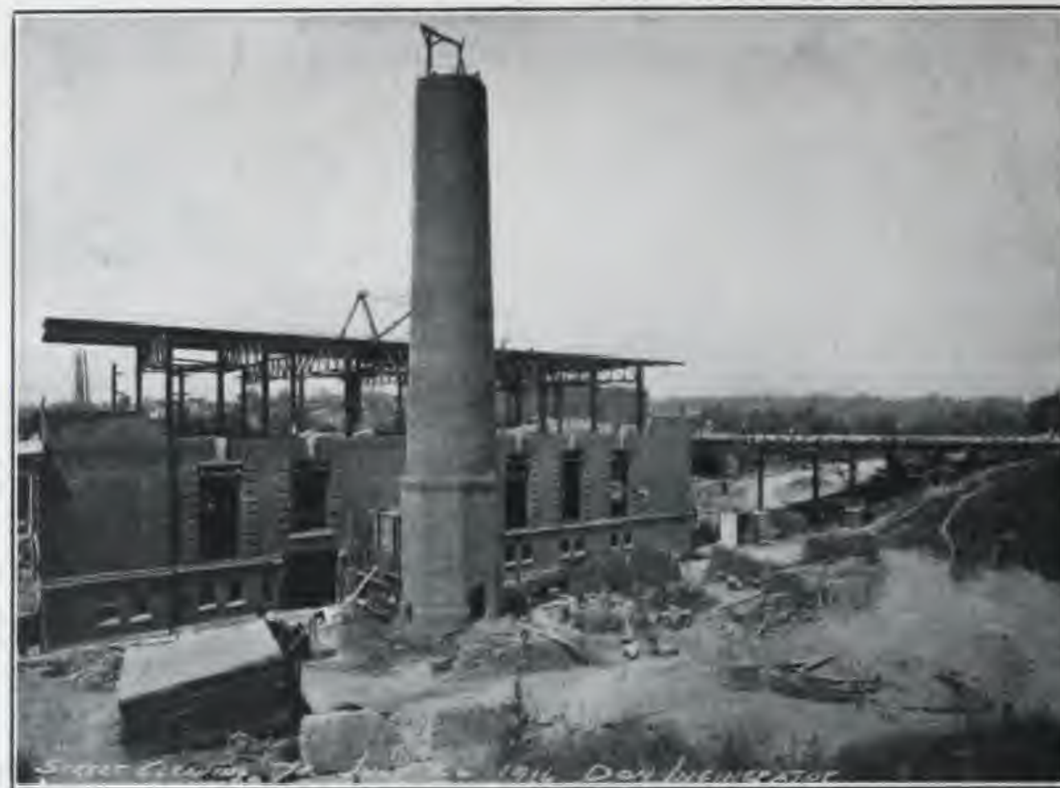
CITY OF TORONTO—DON INCINERATOR. 250 TONS STRUCTURAL STEEL FABRICATED AND ERECTED BY US.
