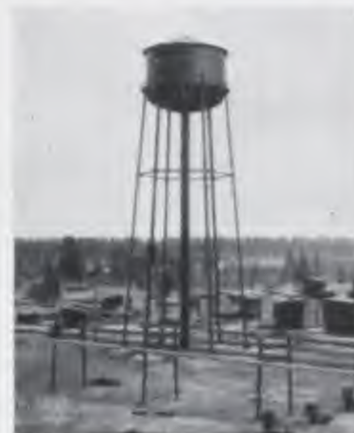
ELEVATED WATER TANK, WESTERN LUMBER MILL.
