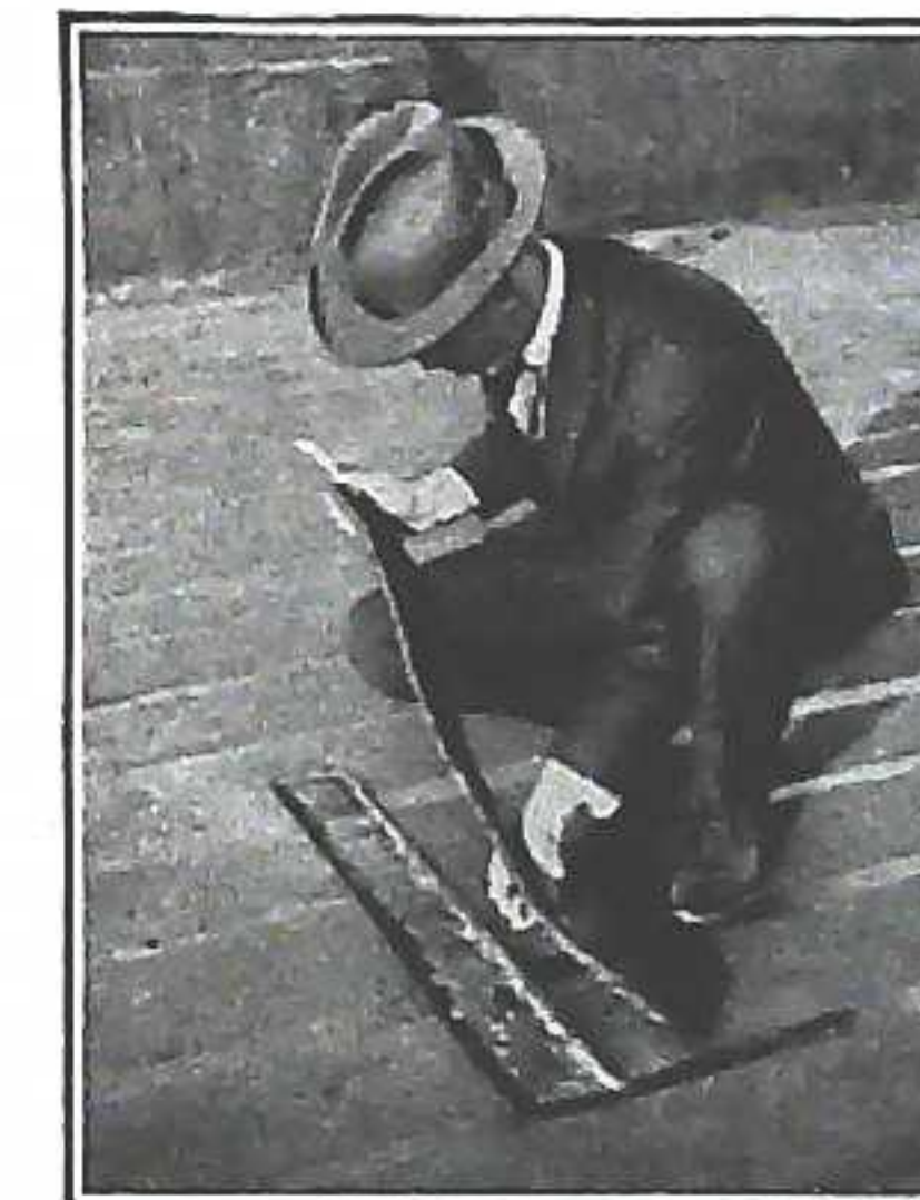
The Barrett Inspector Making the Famous "Cut Test"
