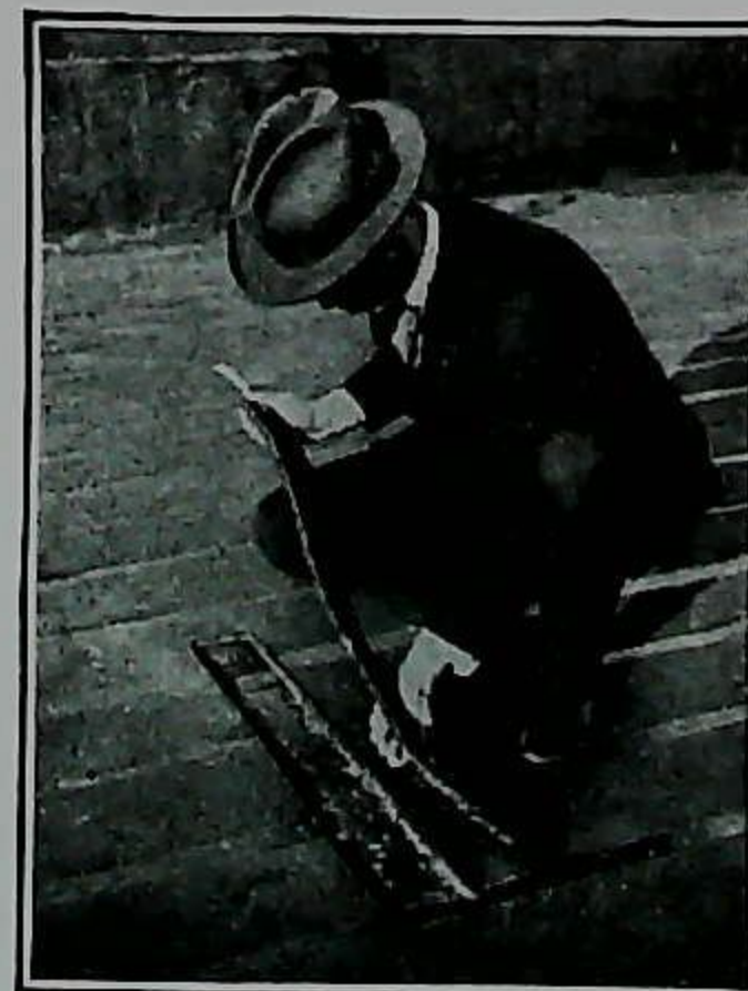
The Barrett Inspector Making the Famous "Cut Test"
