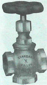
Fig. 314U Cross Valve—Screwed
