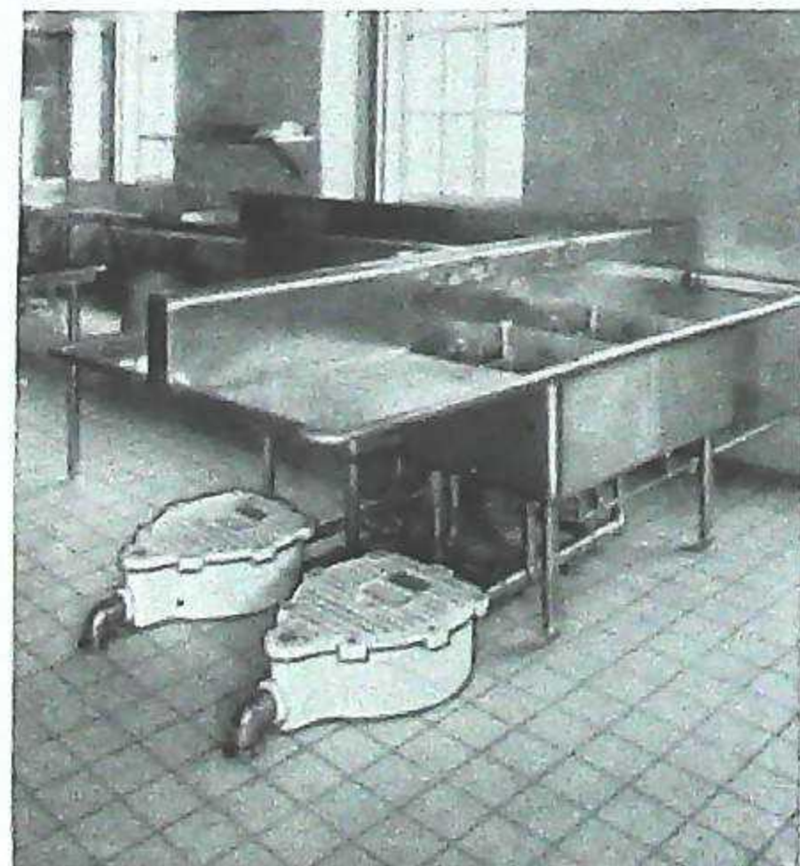
Built-in-the-Floor Installation for Deep Sinks
