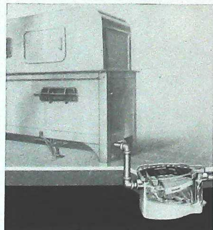
Flush Floor Installation for Electric Dishwasher
